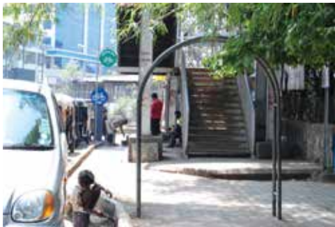
Steps of foot-over-bridge encroaching on cycle track
