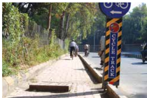
Improperly closed man-hole cover
